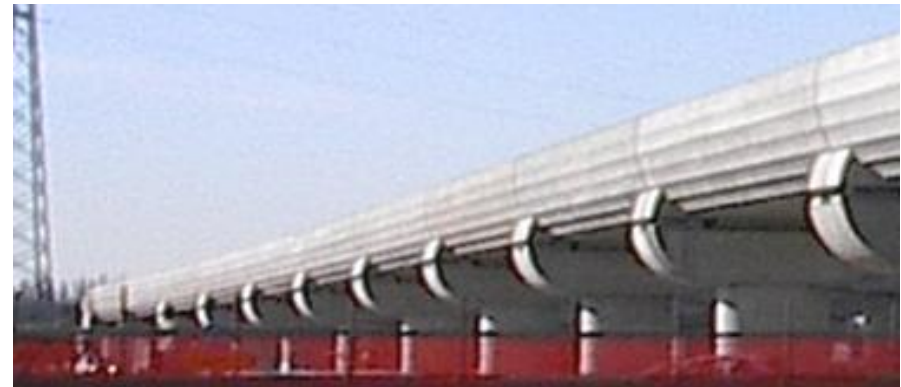
MODENA VIADUCTS, MILANO-BOLOGNA
