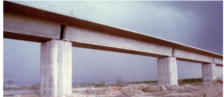
PADULICELLA VIADUCT, ROMA-NAPOLI
