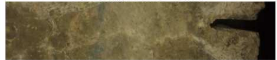
Healed crack after 90 days conditioning (a)
