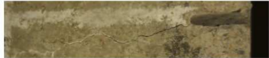
Pre-cracked CMOD 0.6 mm
