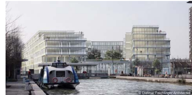
Véolia headquarters, Aubervilliers (93)
