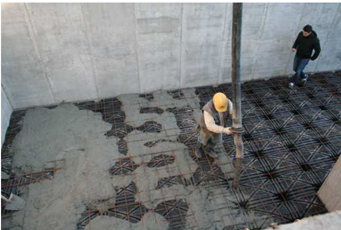
Figure 6. Preliminary casting of the lift-core compartment foundation base: (a) preliminary and (b) final cast / Getto preliminare della fondazione di base del nucleo ascensore.
