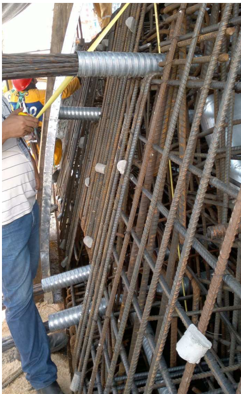
Figura 5. Guaine e cavi trasversali / Ducts and transversal prestressing cables
