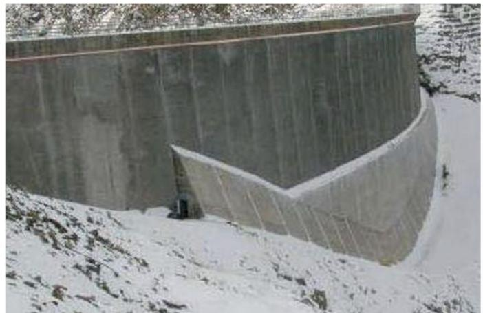
Figure 6. Lago Baitone dam: new concrete upstream face / Diga Lago Baitone (ENEL - BS): nuovo paramento in calcestruzzo, 2008.
