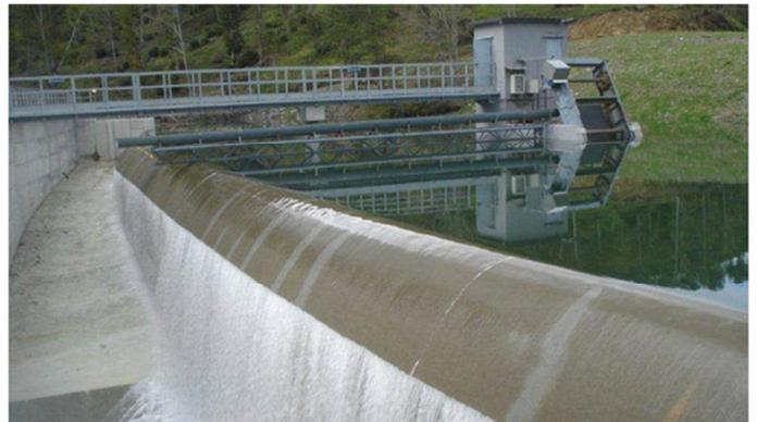
Figure 9. Pian Sapeio dam: reshaping of the spillway / Diga Pian Sapeio (TIRRENO POWER – GE): riprofilatura sfioratori, 2011.
