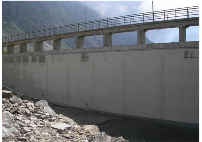
Figure 5. Camposecco dam: PVC geomembrane on the upstream face / Diga Camposecco (ENEL - VB): paramento in geomembrana (PVC), 1991.
