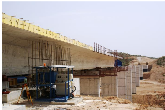
Foto 6 – Centralina elettroidraulica per gestione spinta Picture 6 - Electro-hydraulic control panel for operating jacks
