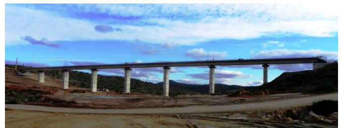
Foto 9 – Vista completa del viadotto ultimato Picture 9 - Overall view of viaduct after completion
