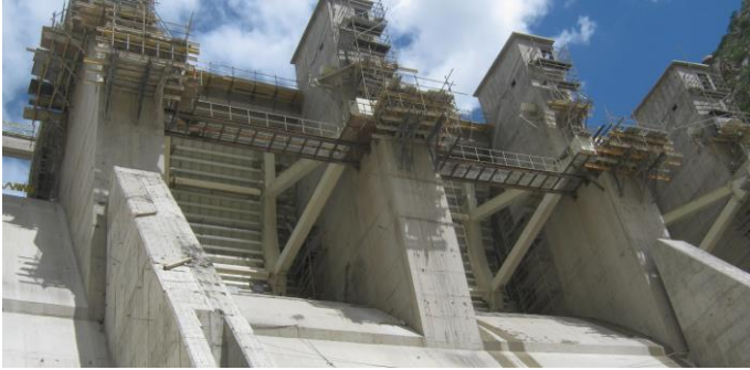
Fig. 17 – Paratoie radiali e flap (lato valle) / Radial gates and flap (downstream side)
