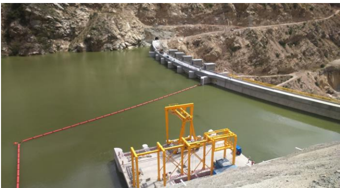
Fig. 19 – Viste generali bacino a quota 1556 m s.l.m. / Overall view of the basin at +1,556 m a.s.l.
