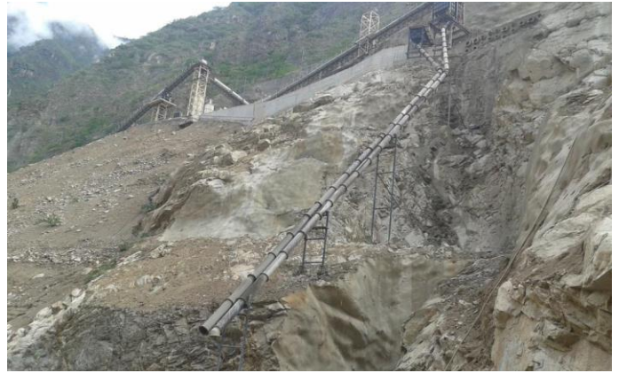
Fig. 6 – Tuberia in acciaio installata a Cerro del Aguila / Steel pipeline at Cerro del Aguila
