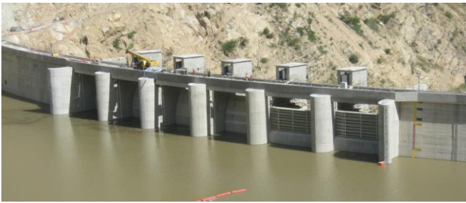
Fig. 18 – Paratoie radiali e flap (lato monte) / Radial gates and flap (upstream side)
