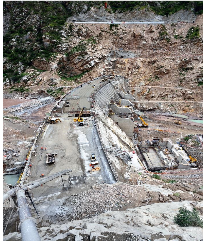
Fig. 10 – Vista durante la costruzione / Top view during the execution of the works
