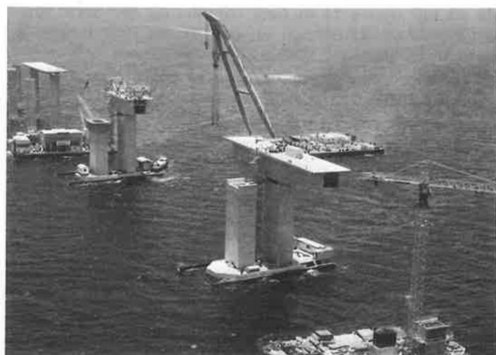
23 - In situ assembly of the 4 m long box section deck segments forming the 3 span continuous girder.
