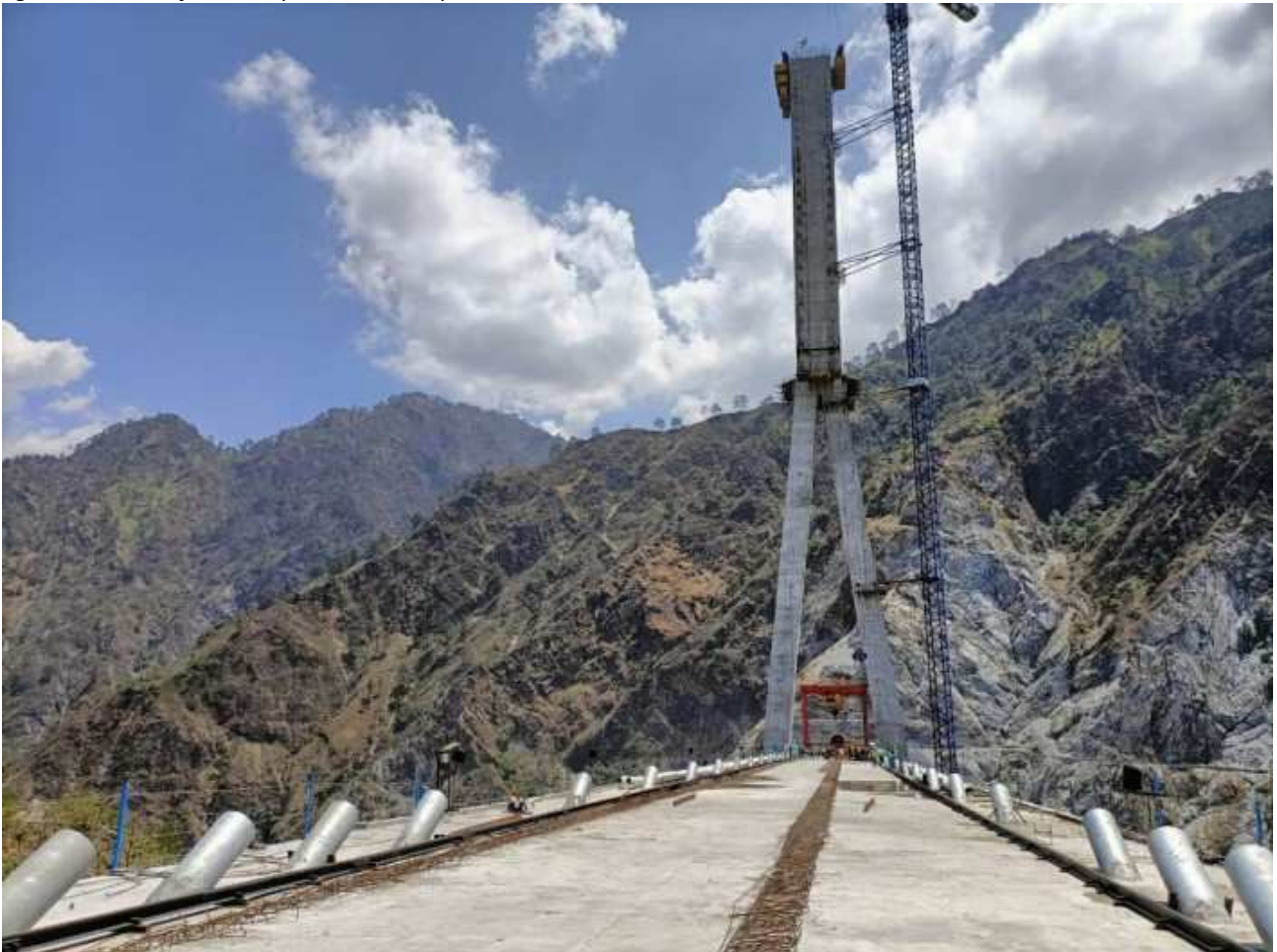
Figure 21. View of the completed lateral span
