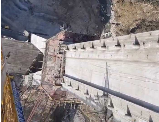
Figure 16. View of the tower from the top
