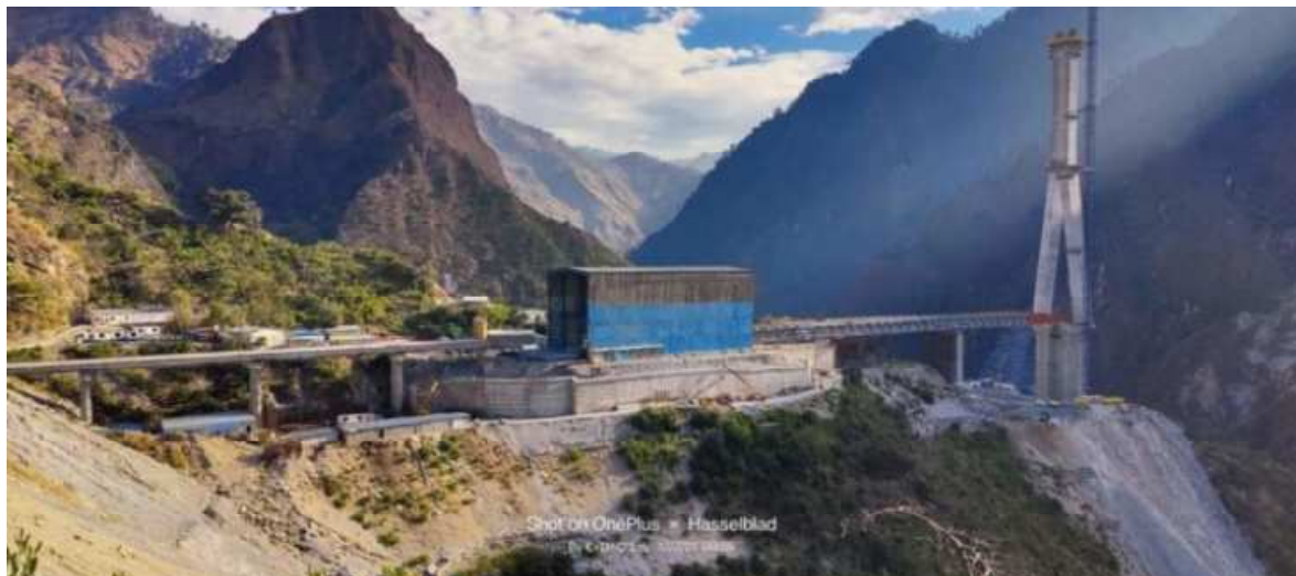
Figure 1. View from Reasi side (right side) of the construction of the Anjikhad Bridge
