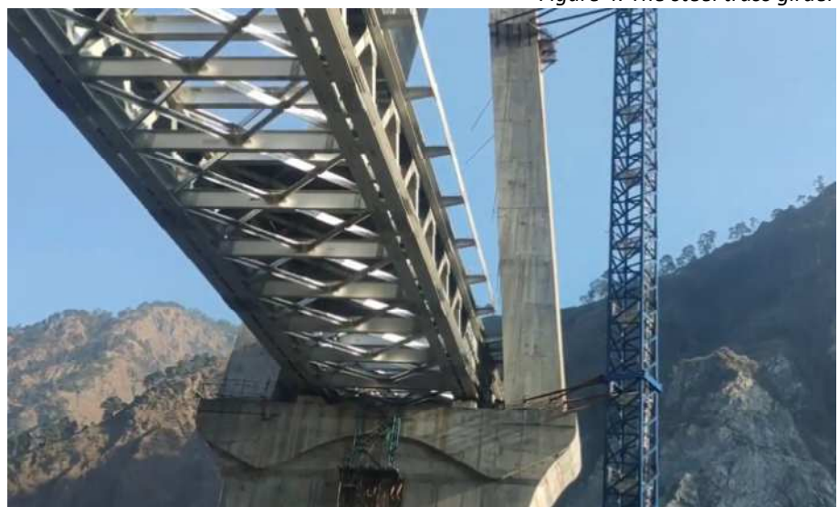
Figure 4. The steel truss girder
