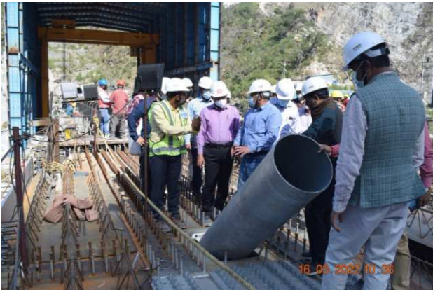
Figure 20. View of one of the stay guide pipe on deck side
