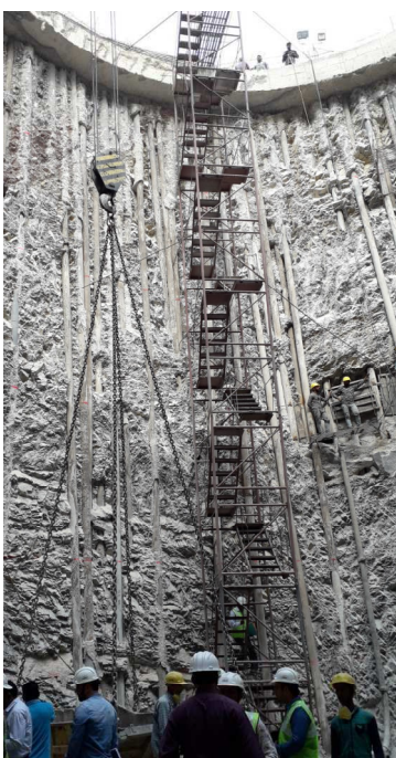
Figure 3. Tower well foundation during the excavation
