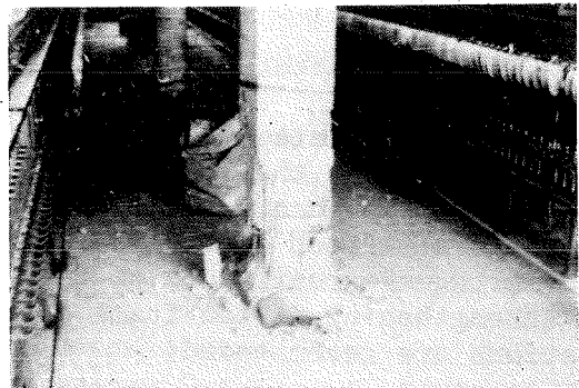
Photo 4 Damage at the bottom part of a column in the top floor.
