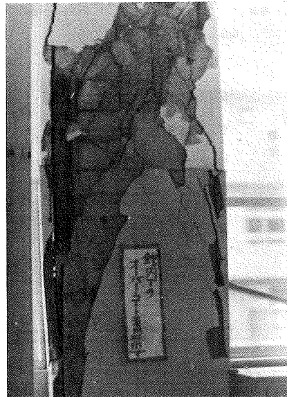
Fig. 3-4 Damaged Pillar (Designed by New Regulations)
