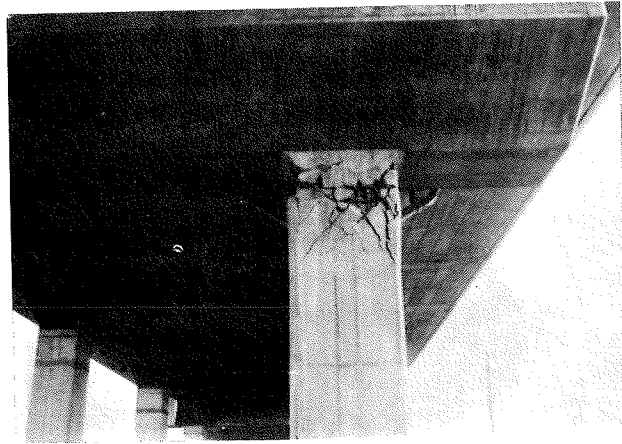
Fig. 2-2 Damage at the Top of Column
