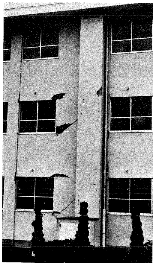
Figure 11 Izumi High School. The two illustrations show, respectively, two sides of a typical building. The rear of the building (left) is relatively open and suffered little apparent damage; damage was heavier on the side with partial-infill wall panels (right). The interior transverse shear walls frame into the columns on the rear but do not frame into the columns on the front because of a longitudinal corridor. All three buildings performed in the same manner.
