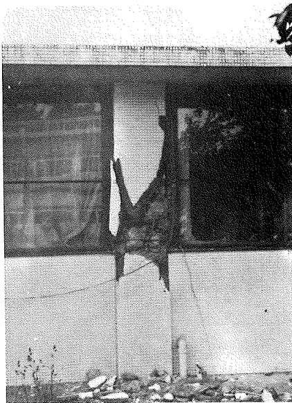
Fig. 3-3 Damaged Pillar (Designed by Old Regulations)
